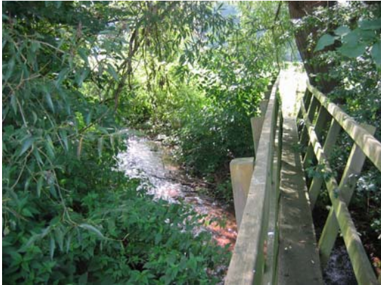
Plate 2: Flow beneath footbridge, south west of Misbourne Farm.
