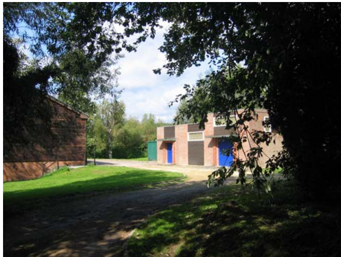
Plate 5: Three Valleys Water Pumping station at Chalfont Mill, Mill Lane.
